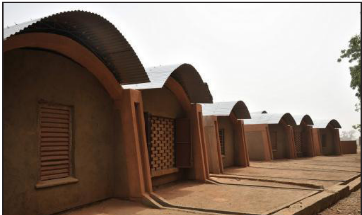
Figure 1: Sustainable housing in Gando, Burkina Faso by Krancis Kere (2011) - uses earth bricks and large roof overhangs for thermal comfort in the houses.
