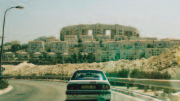
Illegal colony on the West Bank foothills. Typical architecture: larger colonies are built in a fortress fashion.
