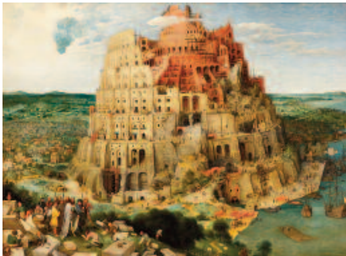
The tower of Babylon. Source: http://www.wallpapergate.com/wallpaper40714.html
