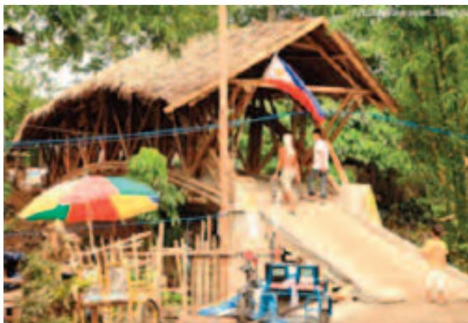
The Matina footbridge in the Philippines, built by bamboo within a project of the Asian Community Architect Network.
