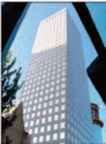
Office building in Vancouver. Photo: Dick Urban Vestbro.
