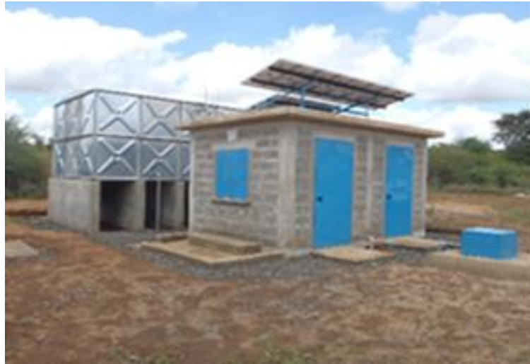
Plate 1.3 A borehole designed to use solar energy but abandoned when the water became yellowish (by Author)
