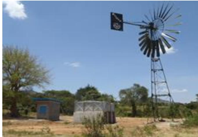
Plate 1.2 A borehole at Makindu designed to use wind power but abandoned when water became yellowish (by Author)
