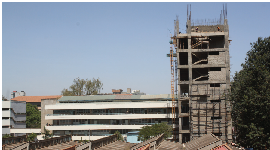
The construction of the S-Block is ongoing. This is expected to provide additional workshop, laboratory and office space for the Faculty of Engineering Sciences and Technology.
