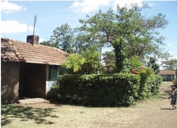
Fig. 7 External view of DU G3 (source: Makachia 2010)
